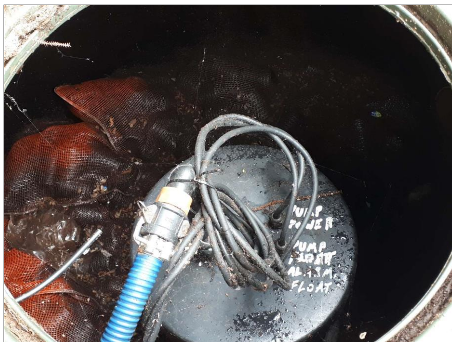
Treatment media inside Biolytix tank
