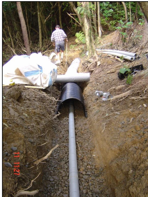
Fig 4: Trench (during construction)
