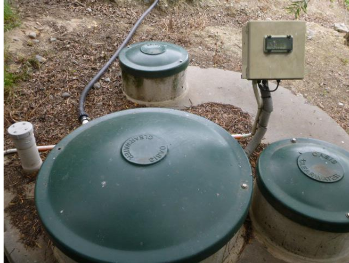
Figure 1: Existing Wastewater System
