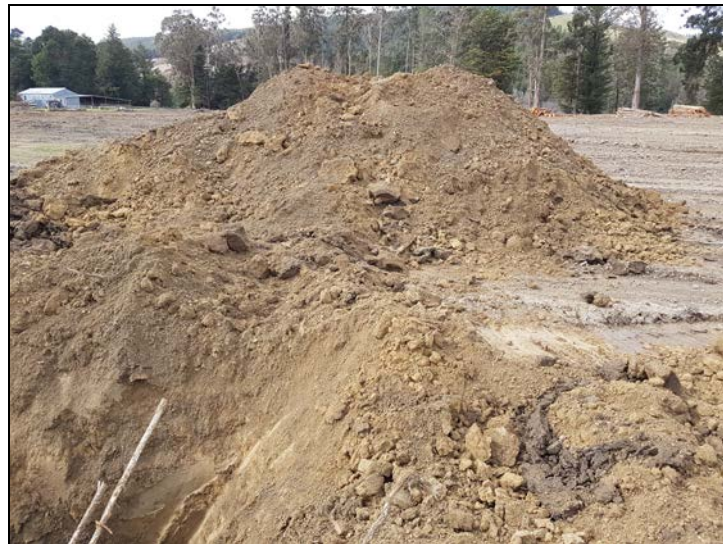
Photo showing material excavated from Test Pit A.
