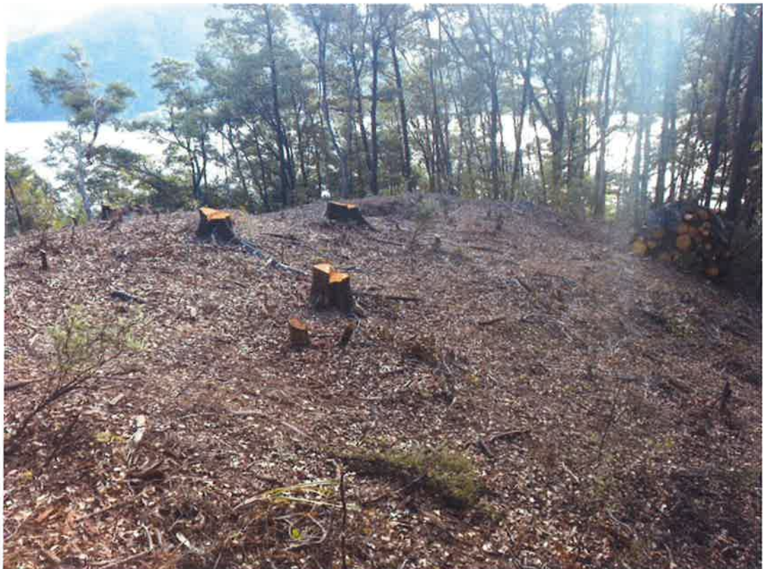
Building site looking north
