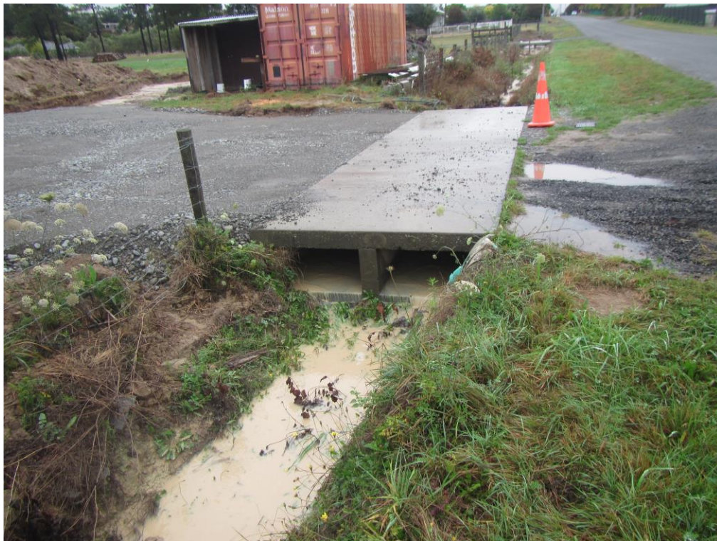
Looking west across the box culvert at the property entrance.
