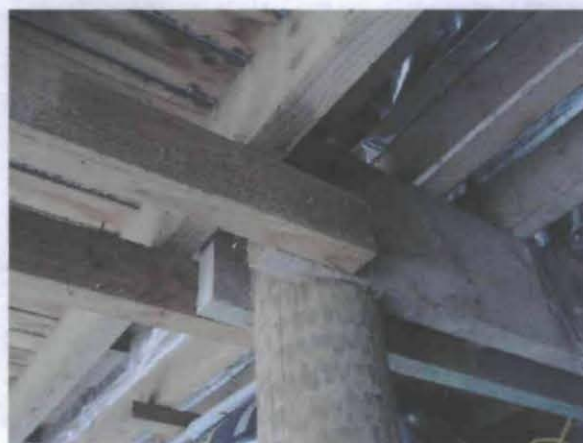
Existing Sub-floor Supports
