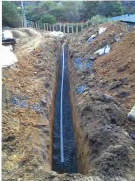
Photograph from contractor – Trench construction
