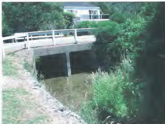
Culvert under Queen Charlotte Drive
