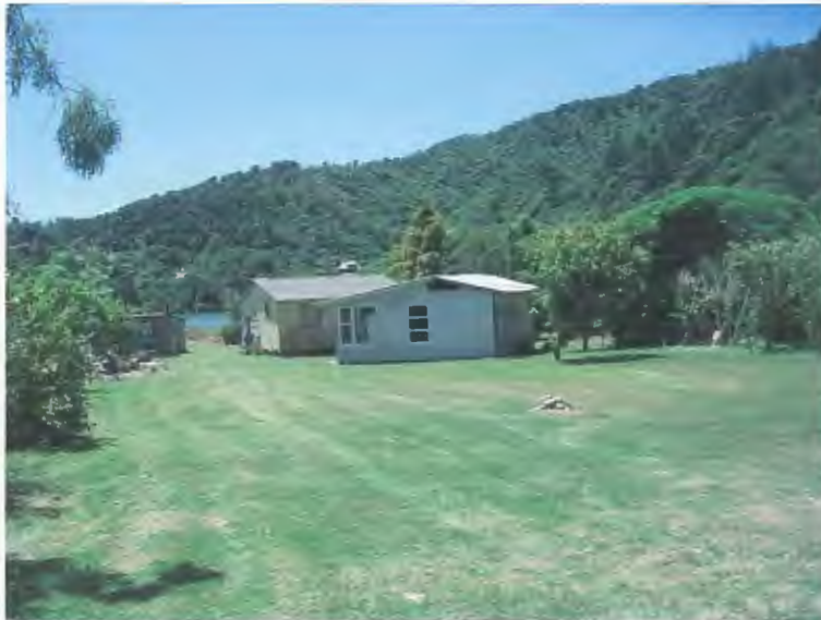
Existing Buildings – Old building at rear to be removed.
