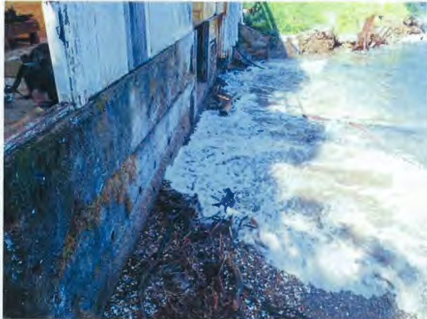
Seawall and wave action at high tide
