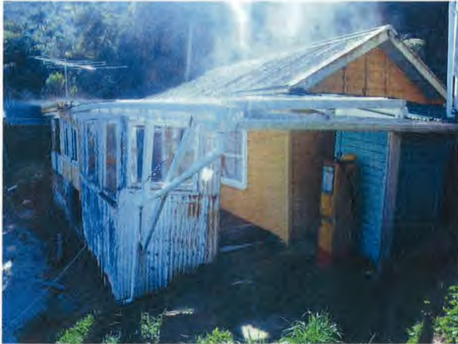
Southern decking and associated wall and roof to be removed
