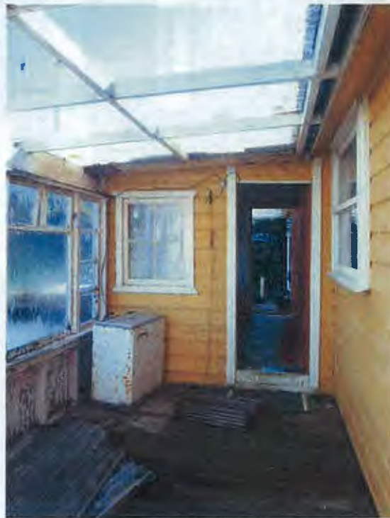
Southern decking area
