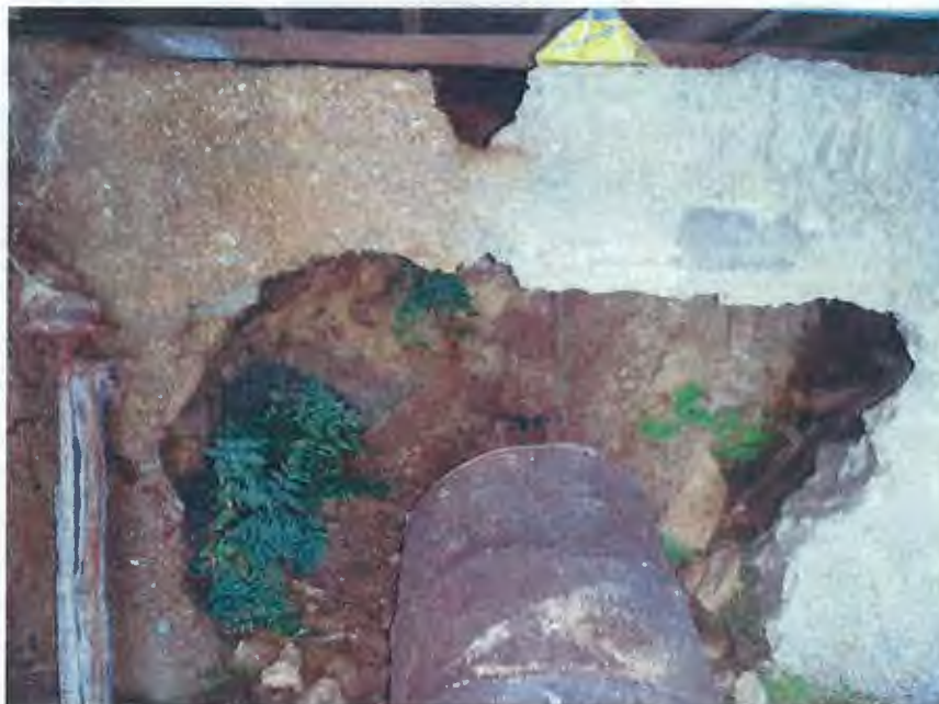
Internal part of seawall
