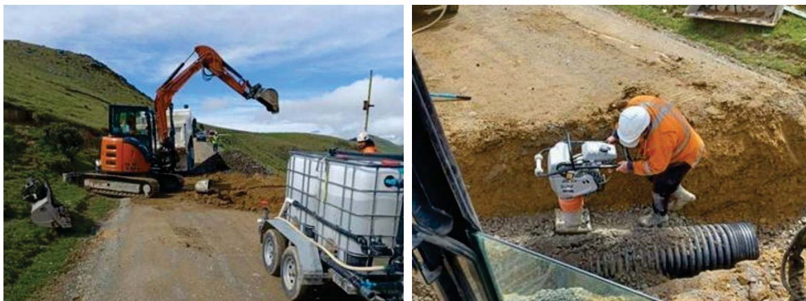
Figure 3-3: Culvert repair works on Croisilles-French Pass Road. (Source: Marlborough Roads Recovery Updates). Similar works will be undertaken in the Port Underwood zone.
