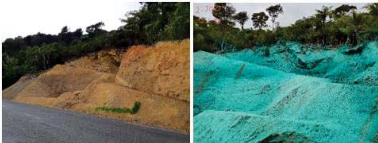
Figure 3-2: Benching, battering and hydroseeding an overslip fault along Queen Charlotte Drive.
